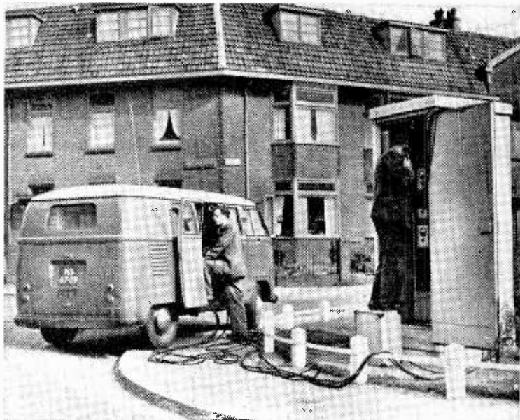
Above: Distribution box for subscribers' lines. Television and/or sound signals can be applied to any subscriber by the insertion of the appropriate resistive or inductive elements which are encapsulated in foamed polyster resin.
